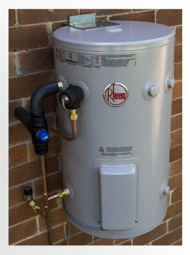
The Rheem Wall Mounting Bracket is a convenient and easy solution to mount a small electric water heater on a wall. The water heater can be mounted on the wall for added safety and to save space.
